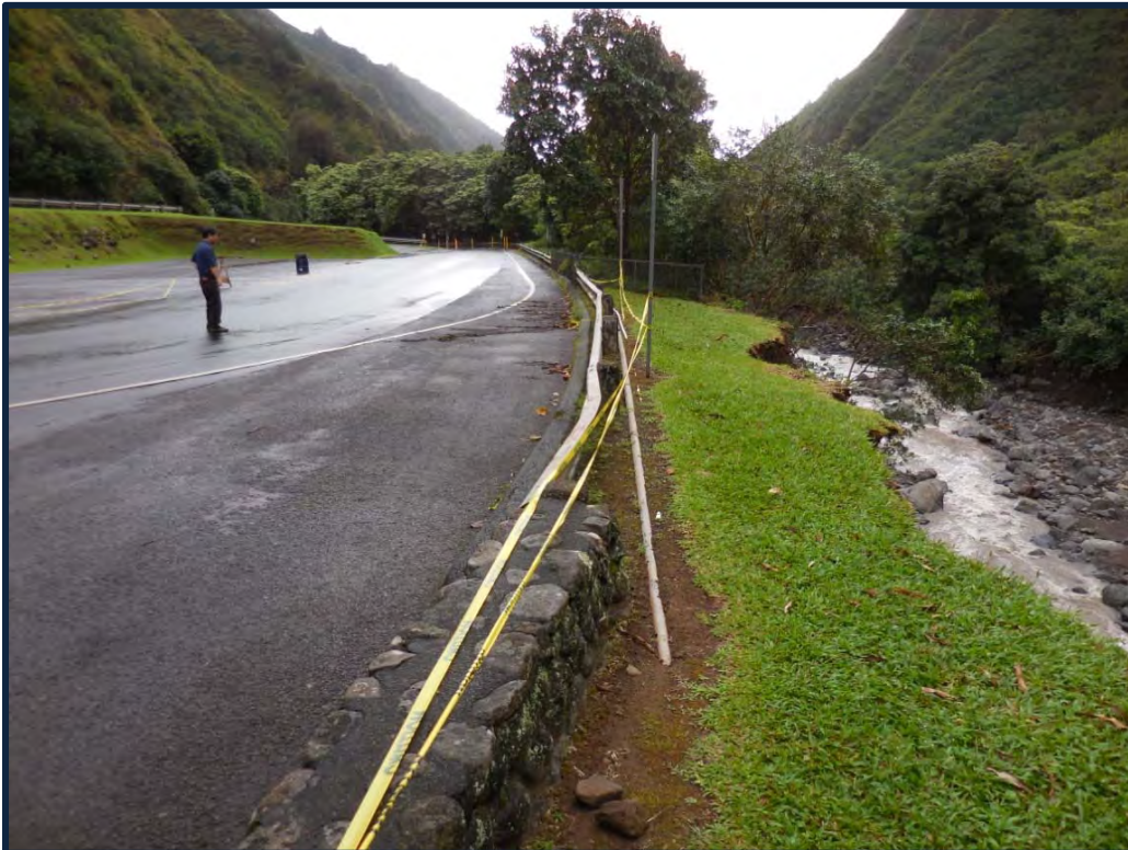
Photograph No. 4: Existing top of slope condition with view in the downstream direction.
