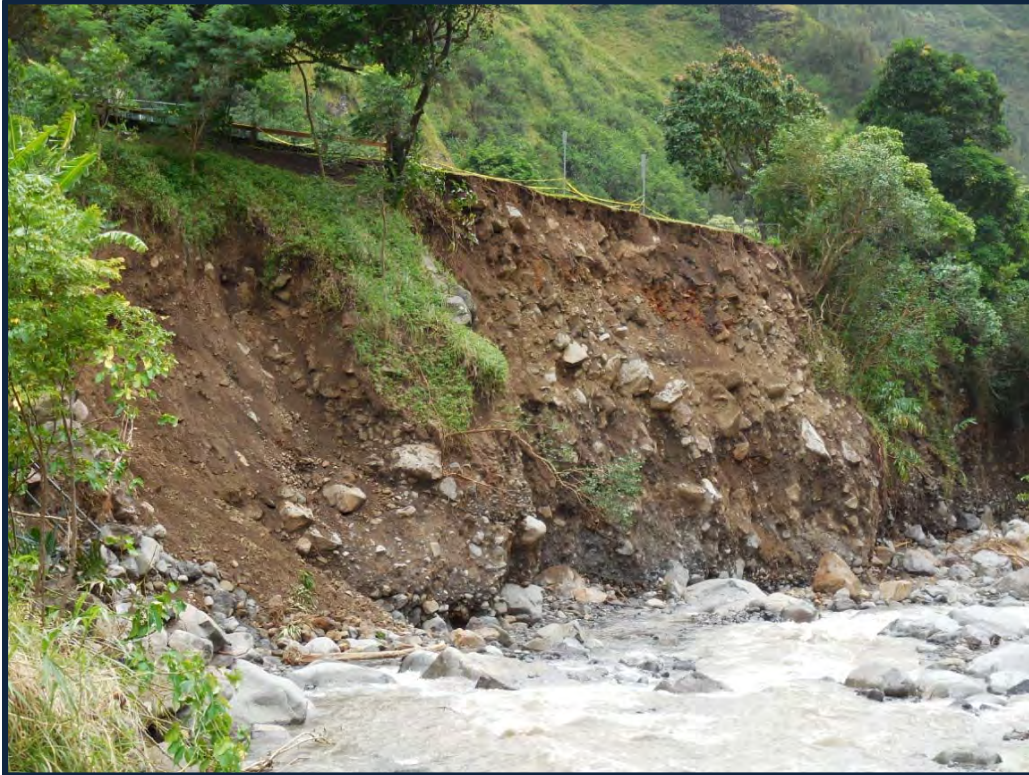
Photograph No. 5: Existing condition of the parking lot slope failure site from the stream elevation. Note the semi-consolidated character of the older colluvial deposits exposed in the lower portion of the slope, in contrast to the overlying unconsolidated overcast fill materials comprising the upper portion of the slope.
