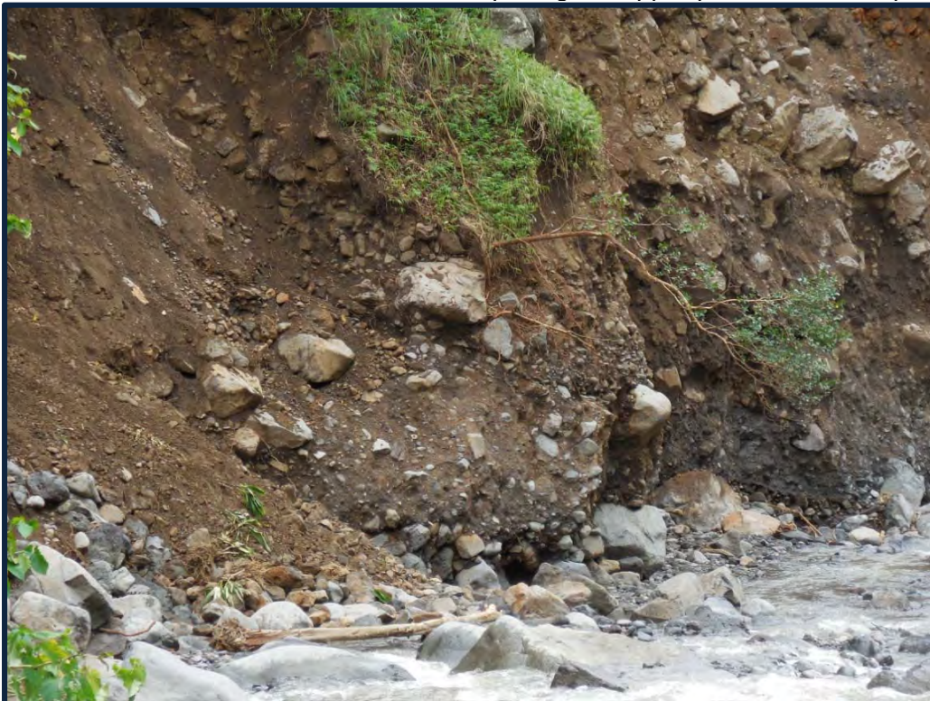
Photograph No. 6: Closer view of the semi-consolidated older colluvial materials comprising the lower slope at the parking lot slope failure site.
