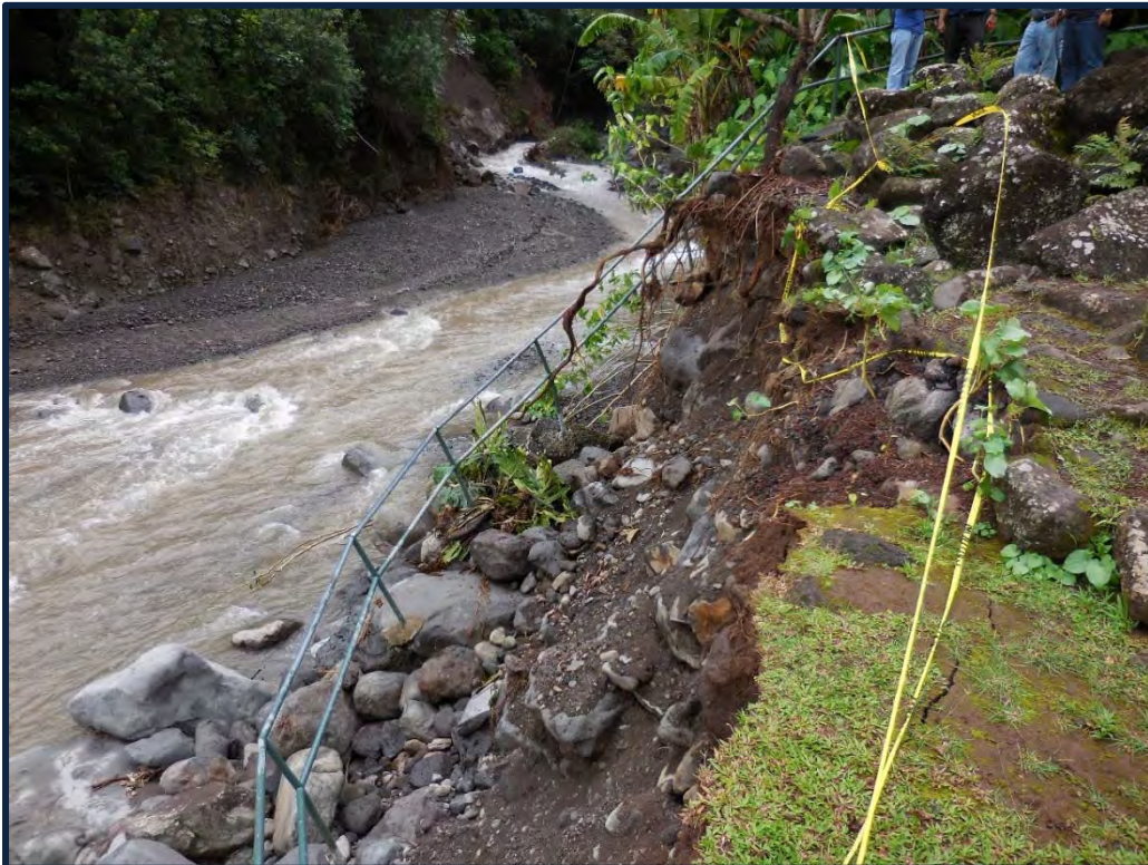
Photograph No. 10: Bank failure and loss of pathway and railings at the short loop trail.
