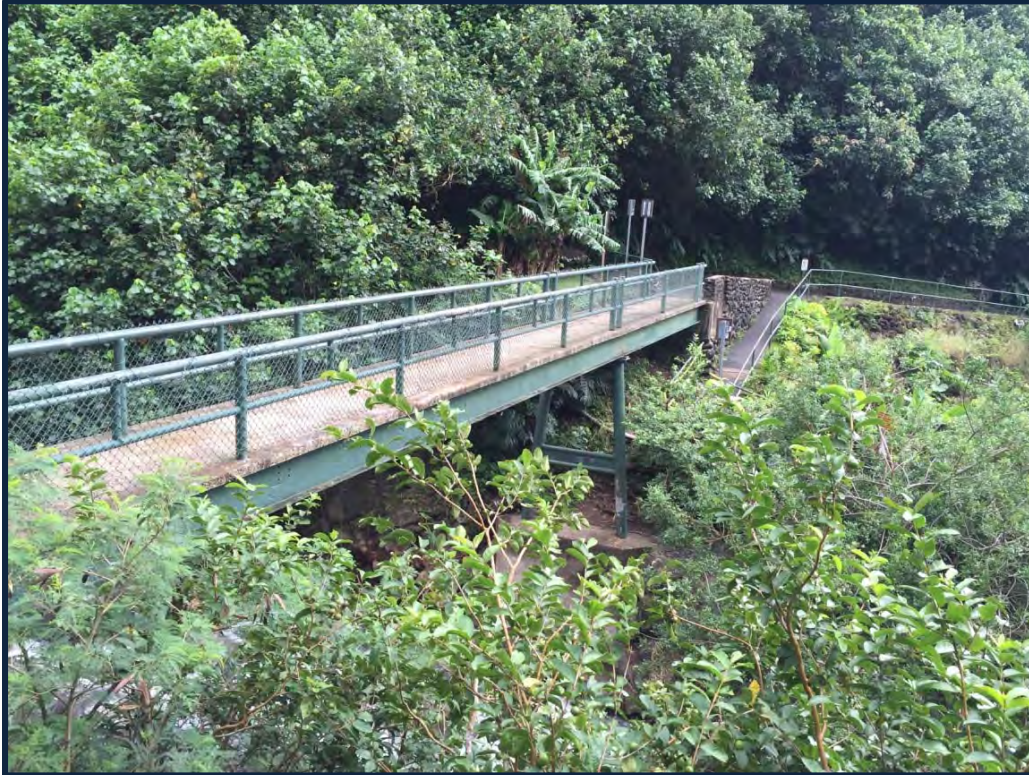
Photograph No. 7: Existing condition of the pedestrian bridge with view towards the north abutment.
