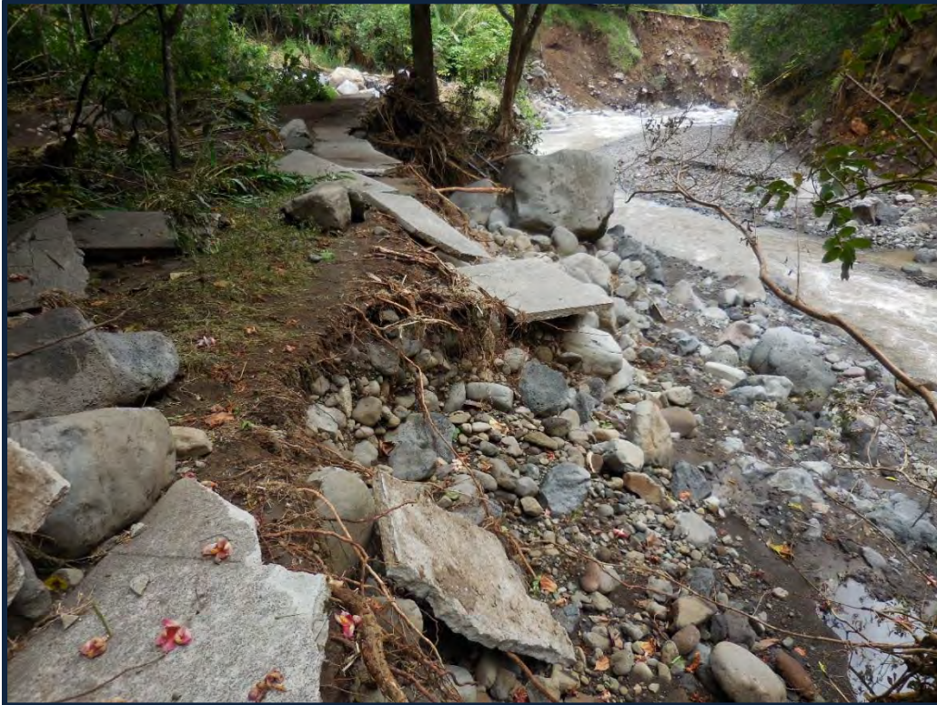
Photograph No. 13: Portion of the concrete pathway on the long loop trail destroyed by floodwater.
