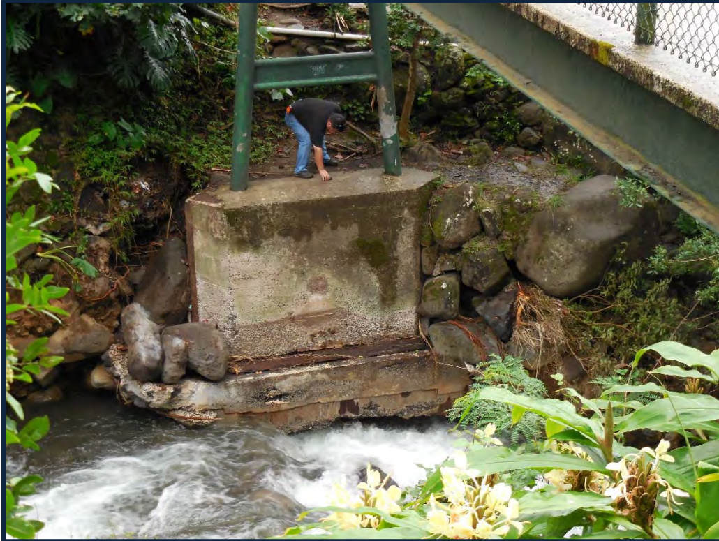
Photograph No. 9: Exposure by stream scour of the existing bridge pier foundation at the northern abutment of the bridge.
