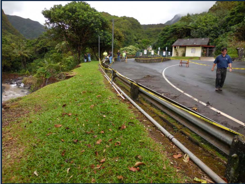
Photograph No. 3: Existing top of slope condition with view in the upstream direction.
