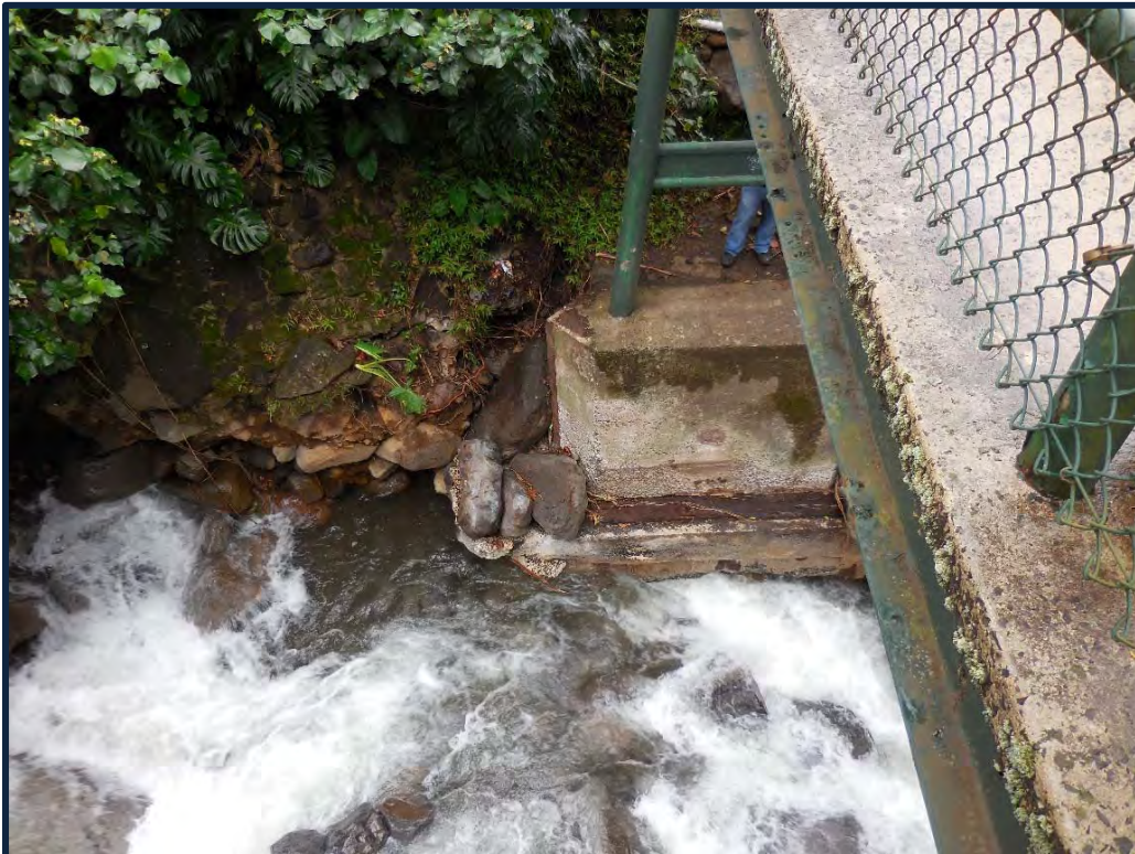
Photograph No. 8: Exposure by stream scour of the existing bridge pier foundation at the north abutment of the bridge.
