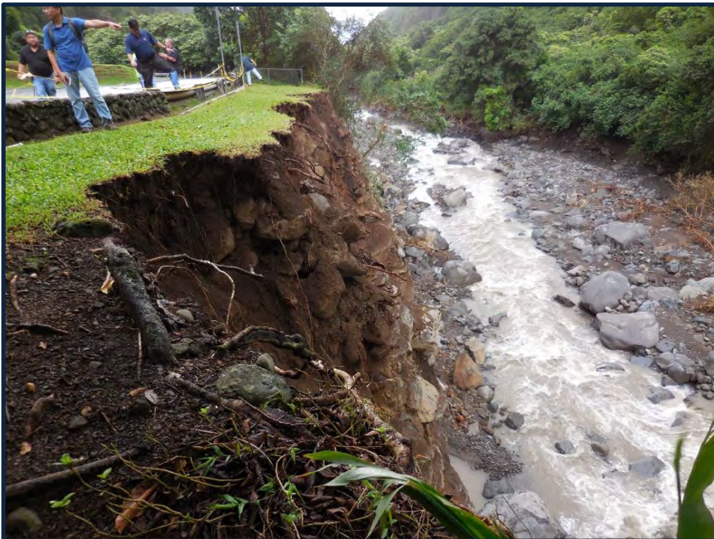
Photograph No. 2: View downstream of the parking lot slope failure site.
