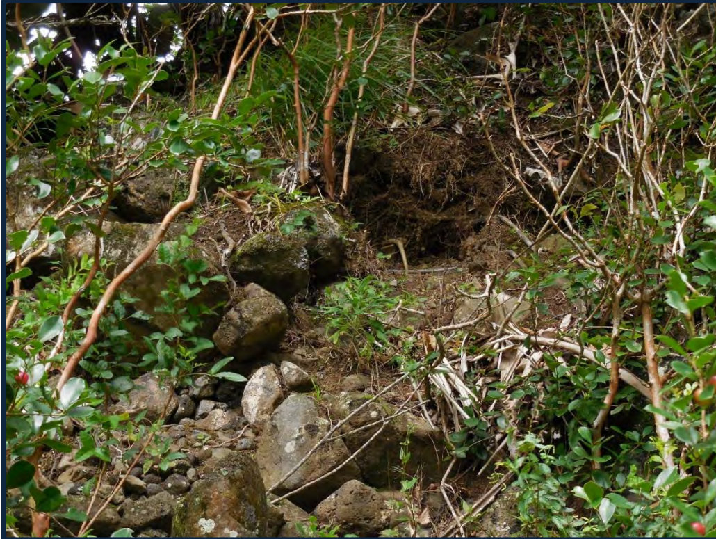
Photograph No. 15: Undermining and exposure of existing basaltic cobbles and boulders mantling the taller slopes adjacent to the pathway. Site of proposed slope scaling.
