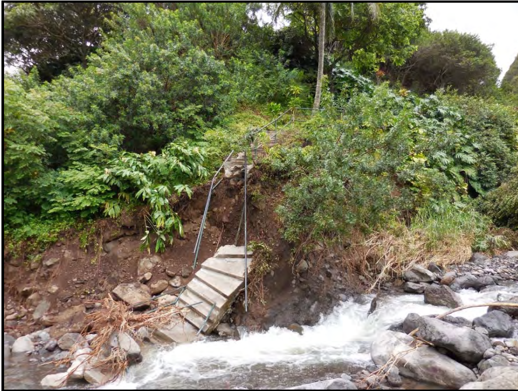
Photograph No. 11: Stream bank collapse truncating the northern portion of the long loop trail.
