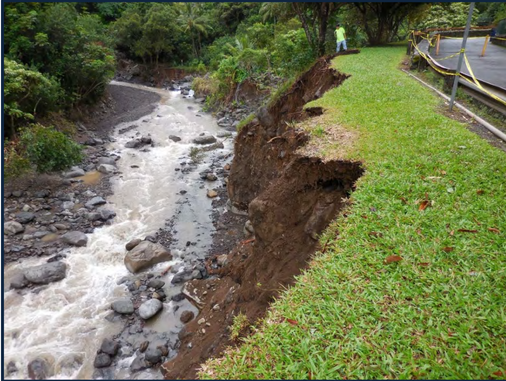
Photograph No. 1: View upstream of the parking lot slope failure site on September 13, 2016
