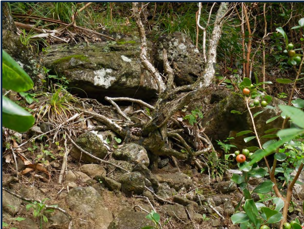
Photograph No. 14: Undermining and exposure of existing basaltic cobbles and boulders mantling the taller slopes adjacent to the pathway. Site of proposed slope scaling.
