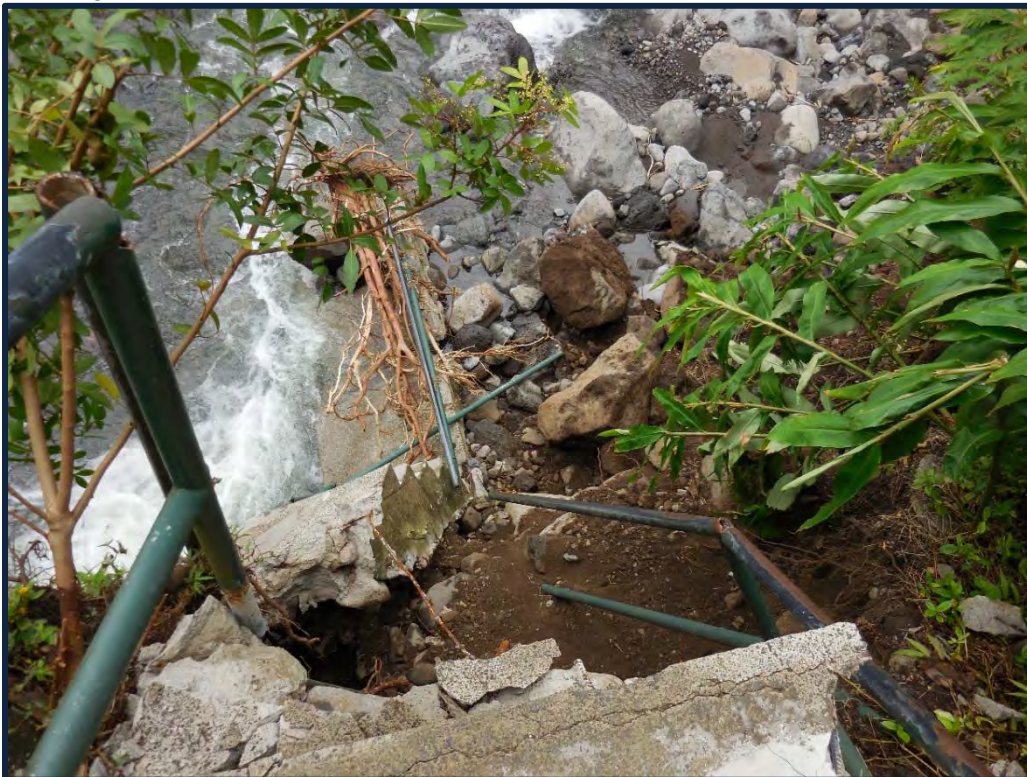
Photograph No. 12: Stream bank collapse truncating the northern portion of the long loop trail.
